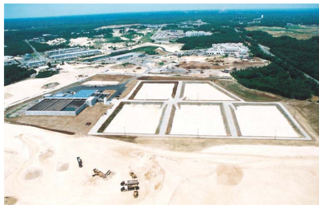
Rapid Infiltration Basins at the Plymouth Wastewater Treatment Plant
