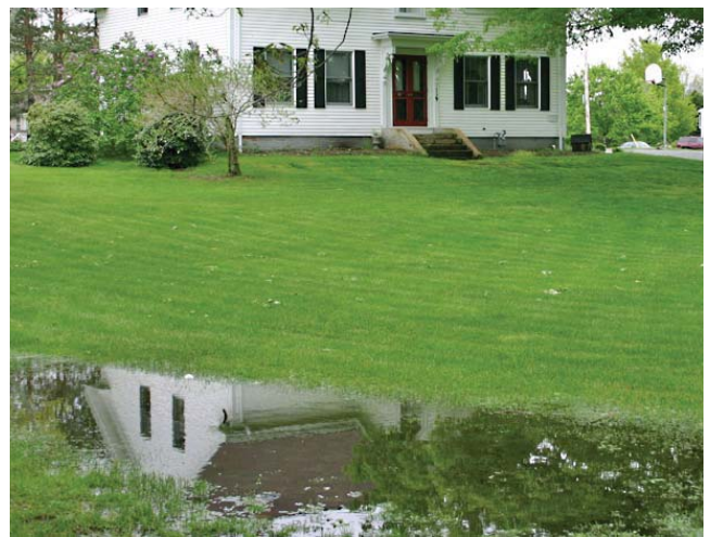
Failed septic tank
